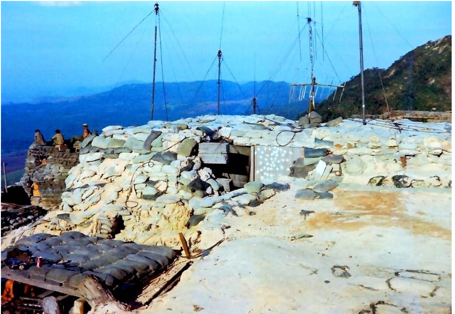
Hill 950 – Hickory Hill – After Jon and his crew fortified the hill.
